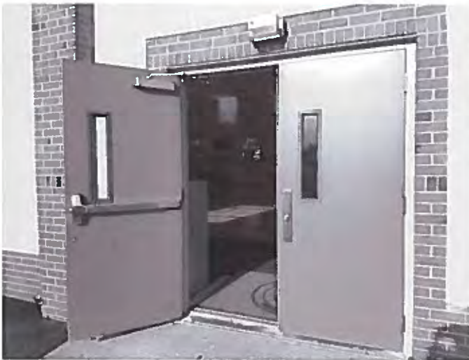
One of our new sets of gym doors.
